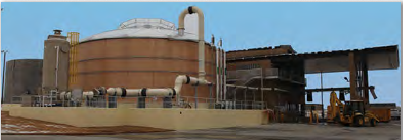
Figure 5.04 - Sludge Dewatering Building
