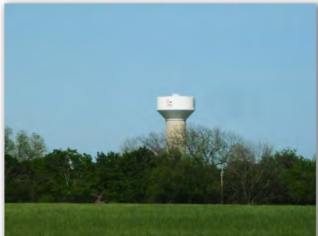
Figure 5.01 - Elevated Storage Tanks
